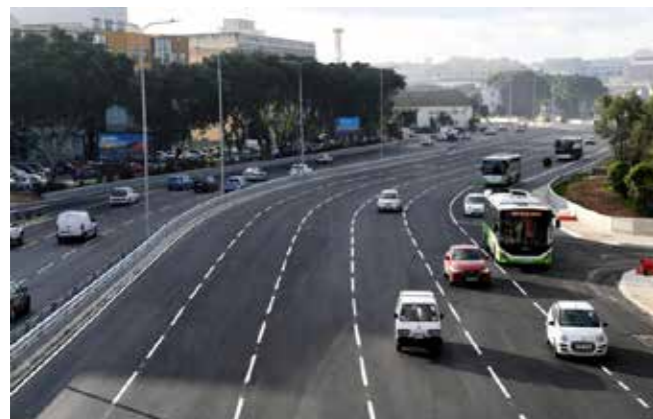
The newly rebuilt Triq Aldo Moro
